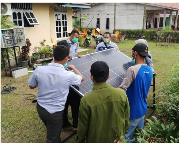
Gambar 4. Proses perawatan panel surya
