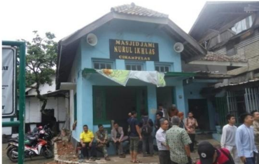
Figure 1. The situation of the Nurul Ikhlas Mosque in 2017
