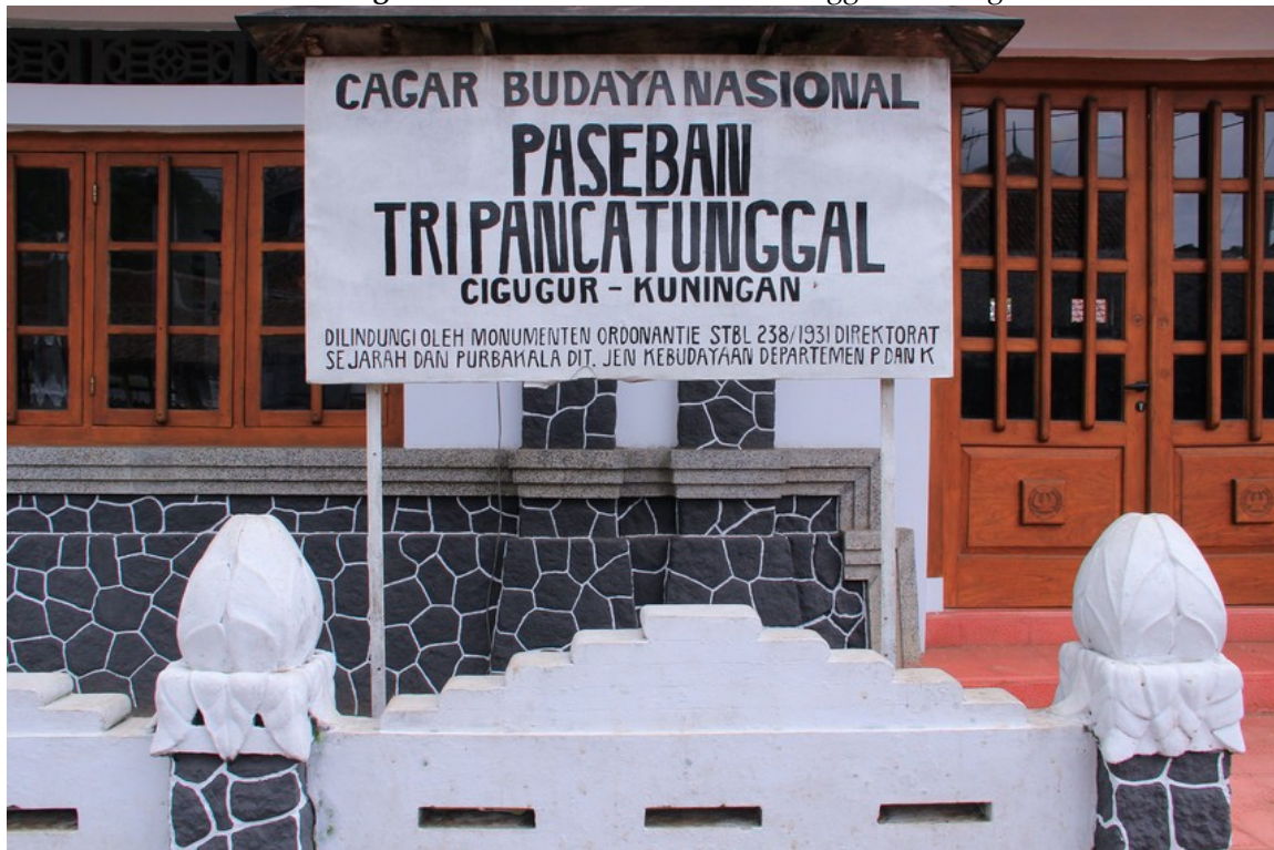
Figure 1. The Paseban Tri Panca Tunggal Building
